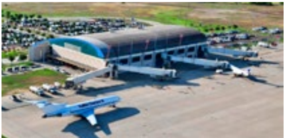
Laredo, TX Laredo International Airport
